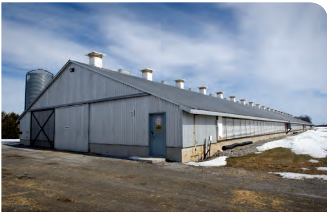
Figure 26. Exterior of a turkey barn.
