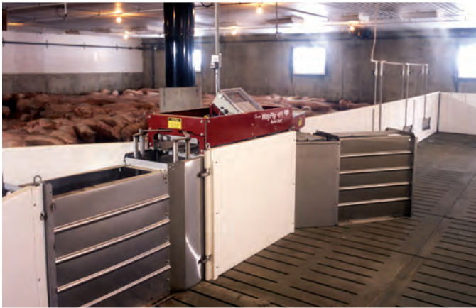
Figure 35. Slatted floor of barn for liquid manure storage under the barn (V5).
