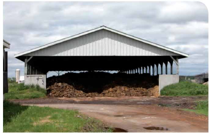
Figure 32. Covered solid manure storage (V2) with slatted walls.
