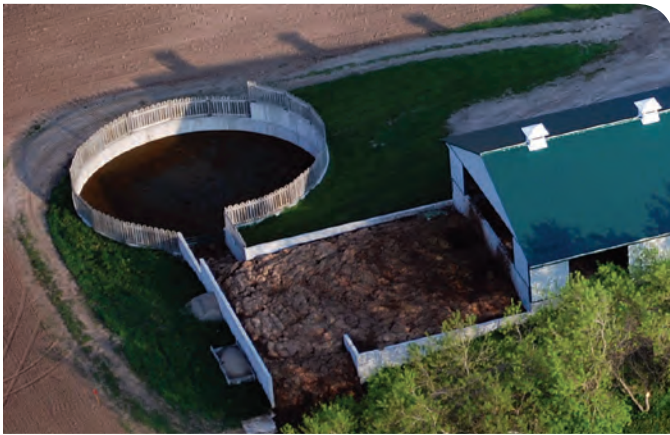
Figure 38. Uncovered liquid runoff storage (L1).
