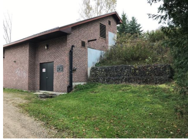
Plate 2. North Pumphouse & Gabions/Slope (view northeast)
