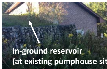
In-ground reservoir (at existing pumphouse site)
